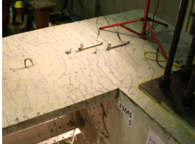
Figure 5-2 Flexural Cracks on Deck of the ESMS Connection
